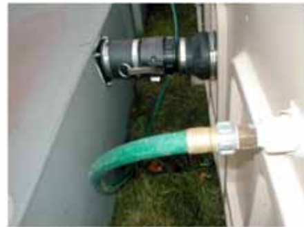
Water and Sewer Connection
