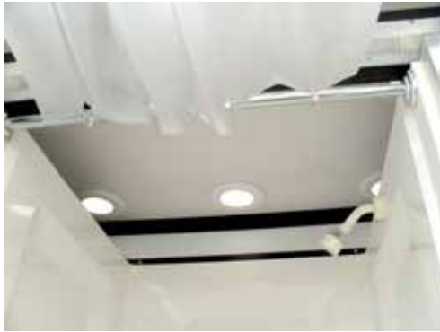
Rear Ceiling/Skylights Shower Head
