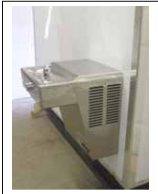
Cold Water Drinking Fountain
